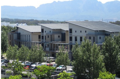
CIMSO Cape Town Offices, South Africa
